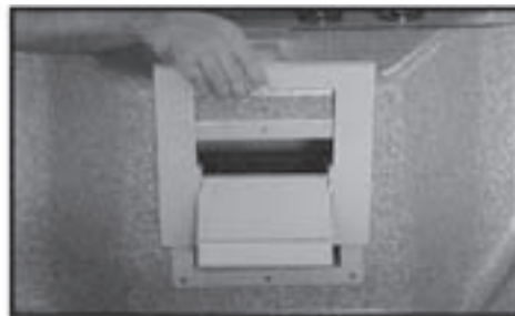
2. Remove Front Filter Plate
