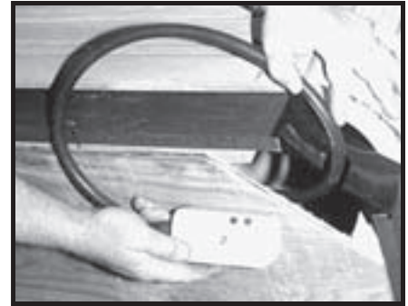
Ground fault interrupter plug & power cord fished through arched corner of the spa
